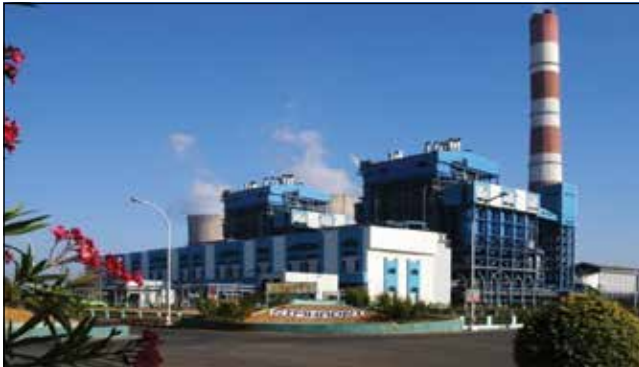
Simhadri Power Project of NTPC, Visakhapatnam district (A.P.)
