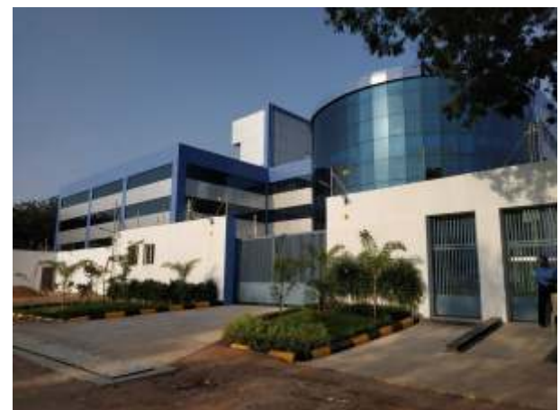
A view of Data Centre at Hyderabad
